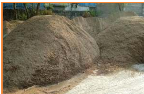
Fig 14: Sand produced from C&D Waste is utilised in the RMC Plant of Nuvoco Vistas Corp. Limited
