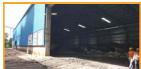
Fig 10: AFR Storage facility at Orient
