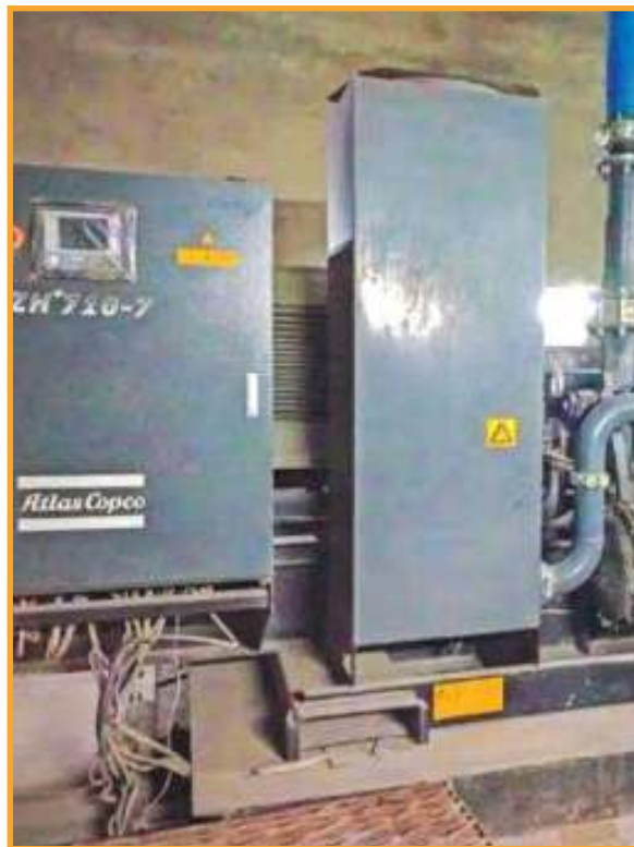
Fig 3: Centrifugal Compressor in place of Reciprocating Compressor modification
