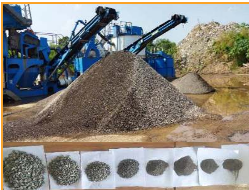
Fig 13: Aggregates and Sand from Construction & Demolition
